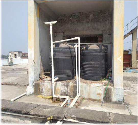
Construction of tanks and bunds
