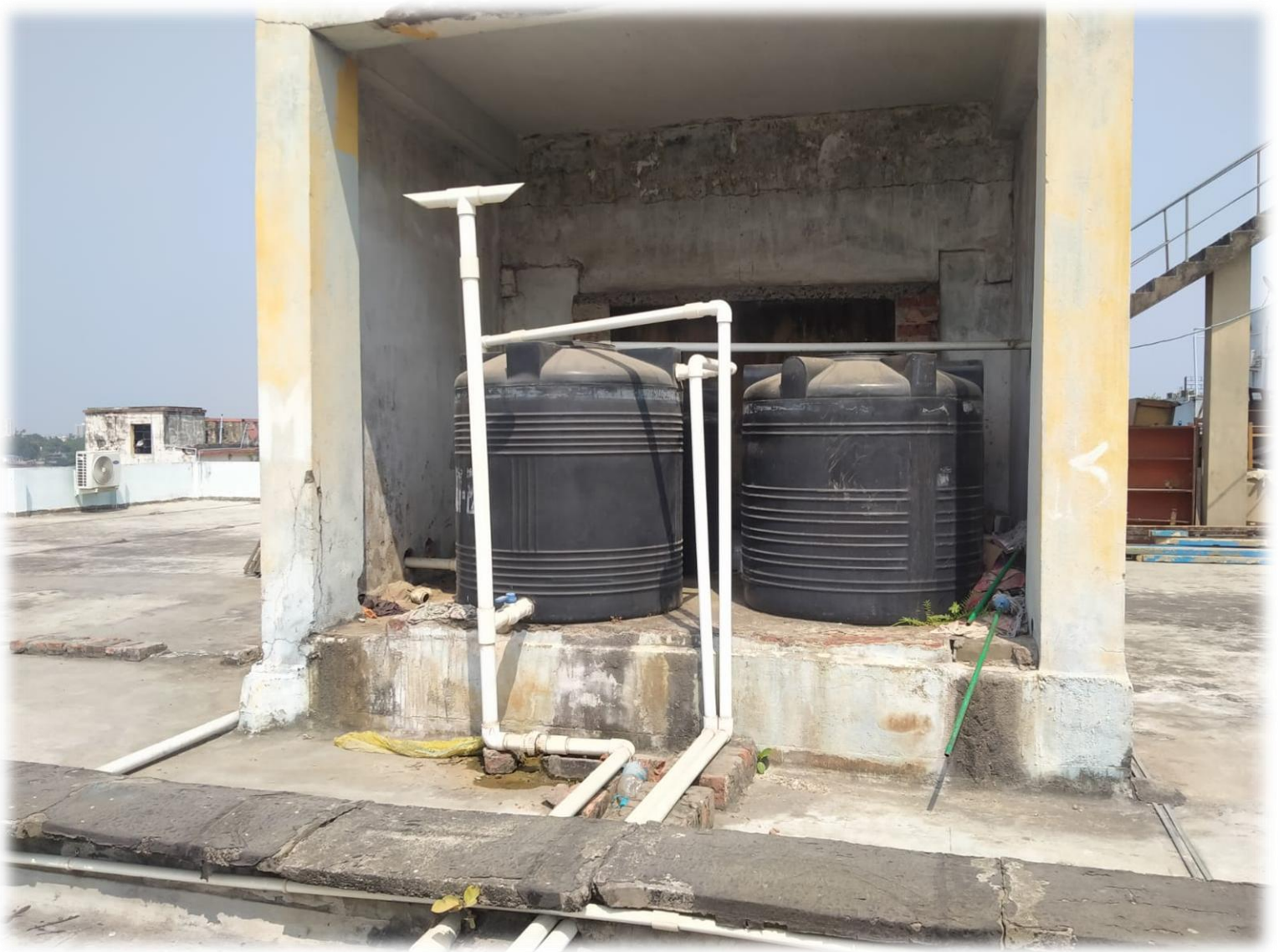
Construction of tanks and bunds
